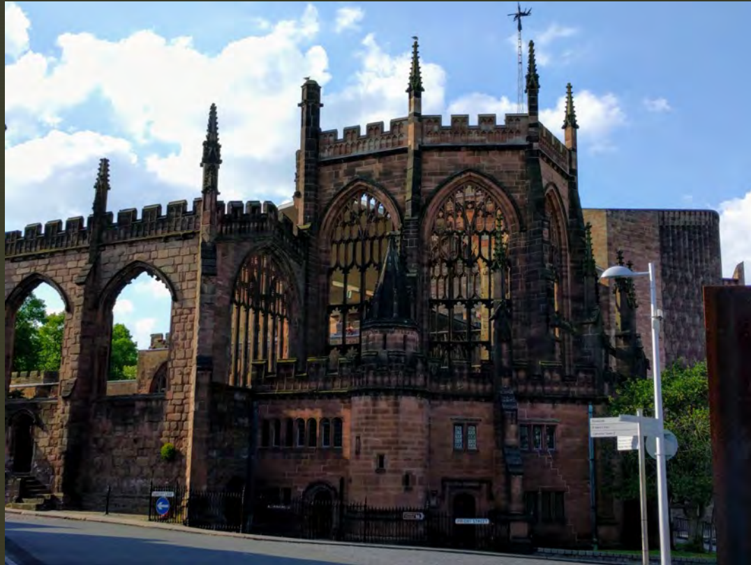
The bombed out cathedral shell is joined to modern construction
